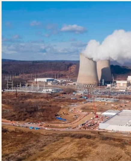
An Amazon Web Services data centre, foreground, under construction in Pennsylvania in January 2024 © Ted Shaffner
