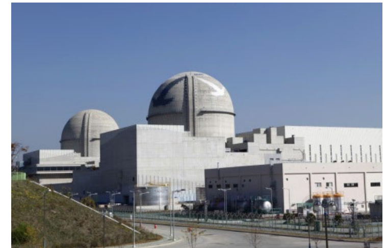
APR-1400 (KEPCO) in Barakah (UAE), 4 x 1400 MW 5'000-8'000 $/kW installed, construction time 5-8 y, LCOE <100 $/MWh
