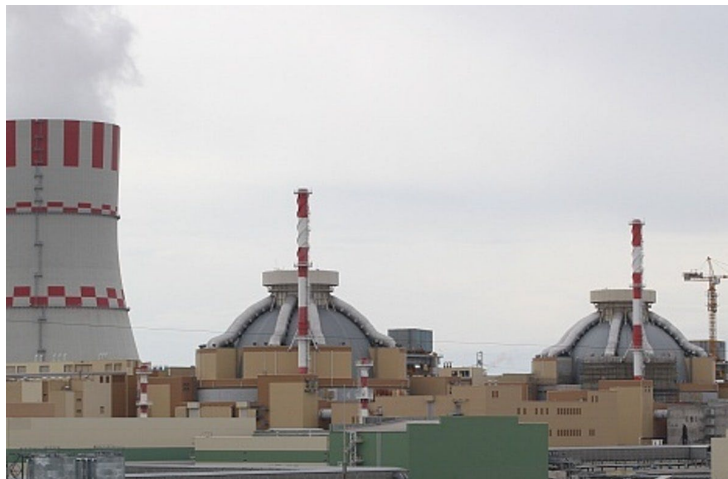
VVER-1200 (Rosatom) in Tianwan (China), 2 x 1250 MW 5'000 $/kW installed, construction time 5.5y, LCOE <70 $/MWh
