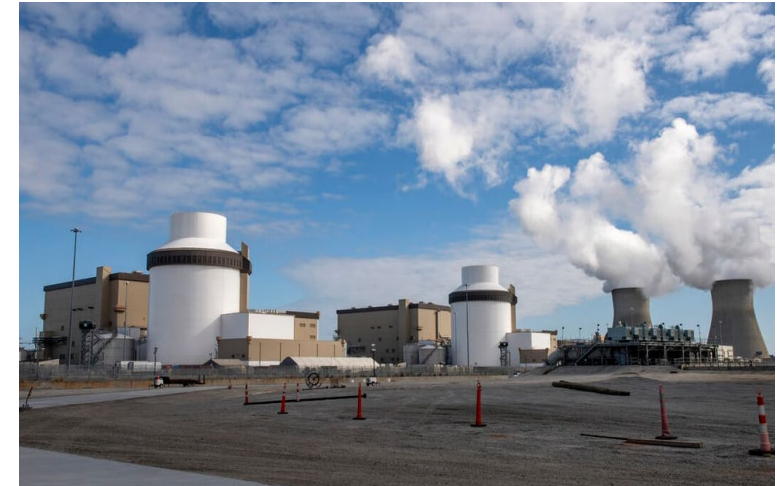
AP-1000 (Westinghouse) in Vogtle (USA), 2 x 1200 MW 9'000 $/kW installed, construction time 10y, LCOE >150 $/MWh
